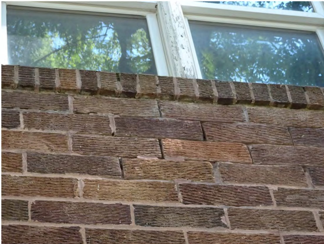
Needed Repairs – Tuck-Pointing, Window Frame Painting / Sealing
