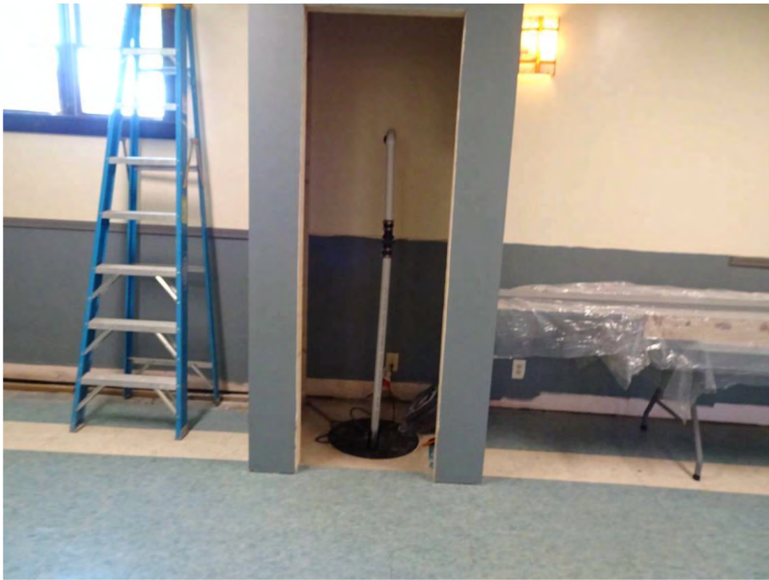
Newly Installed Sump Pump
