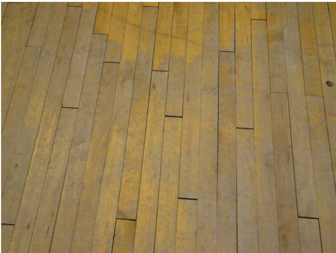
Hardwood Floor Needing Re-Finishing
