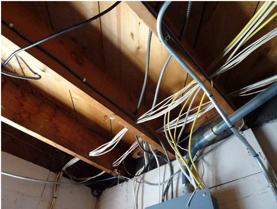
Excessive Joist Penetrations – Back of House First Floor
