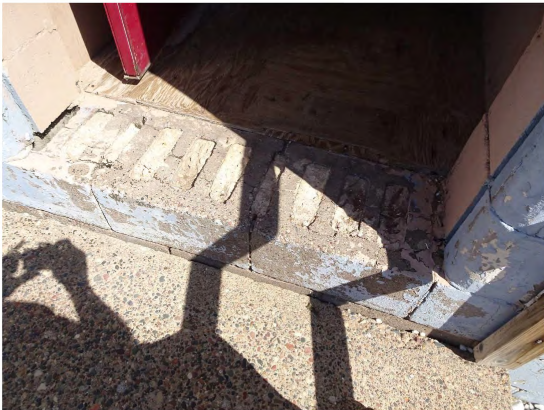
Exterior View – Back Exit Door Step / Threshold Needing Repairs
