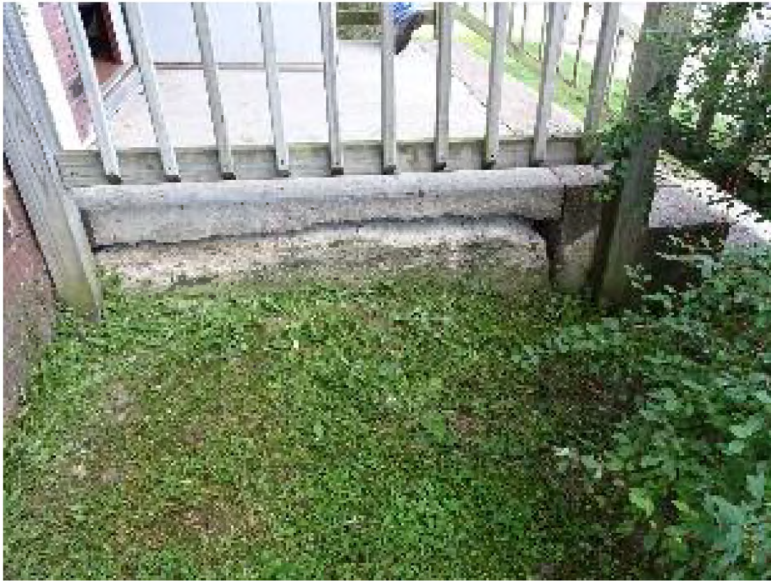
Front Stair Degradation
