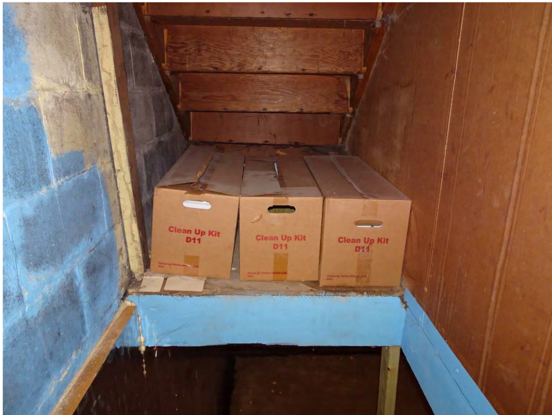
Interior View – Non-Rated Stair with Combustible Storage Beneath
