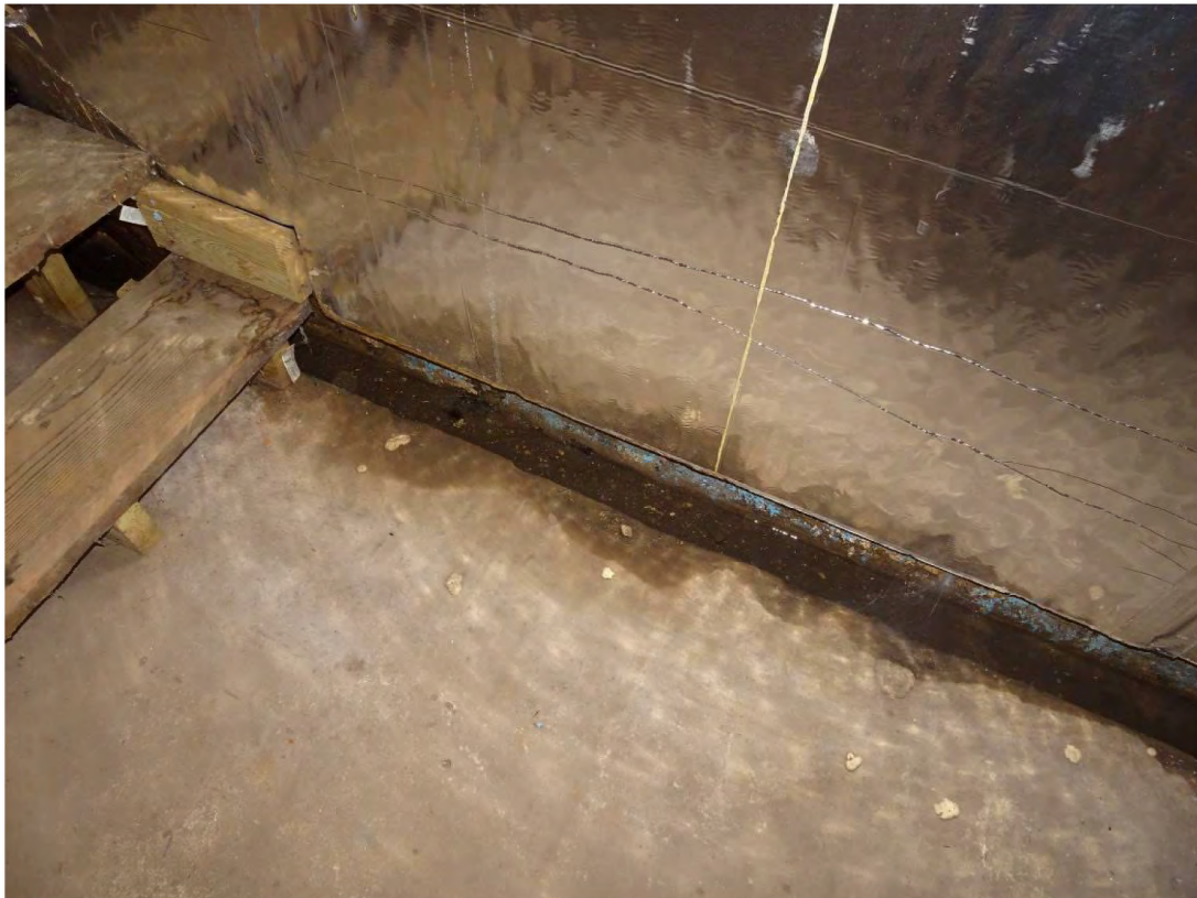
Interior View – Basement Perimeter Seepage Drainage Trench
