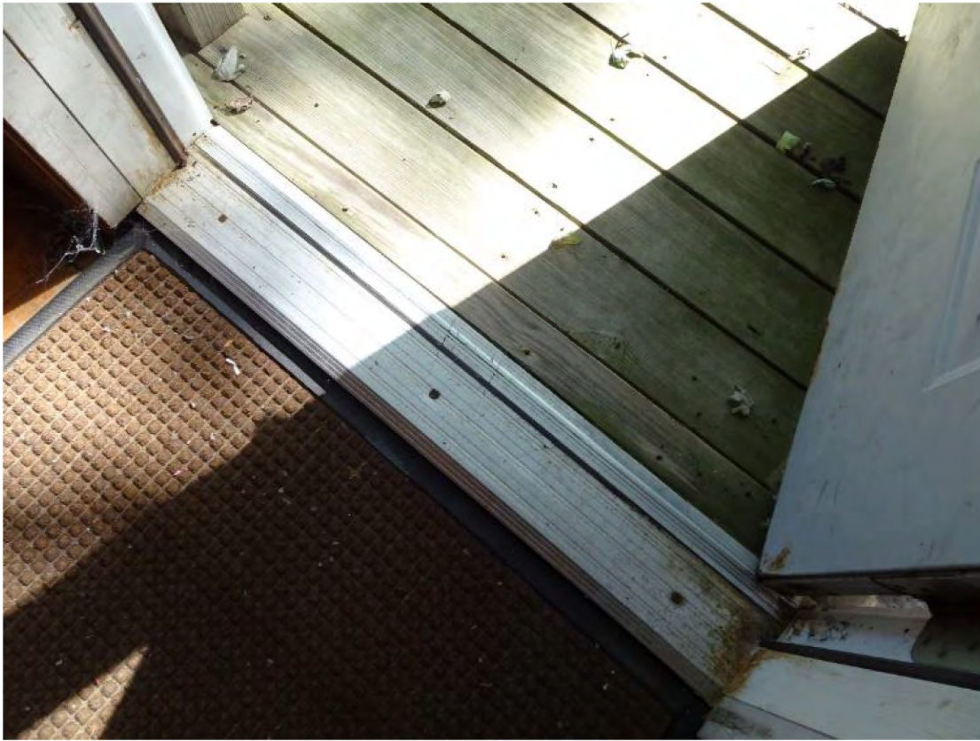
Non-Accessible Ramp Entry Threshold
