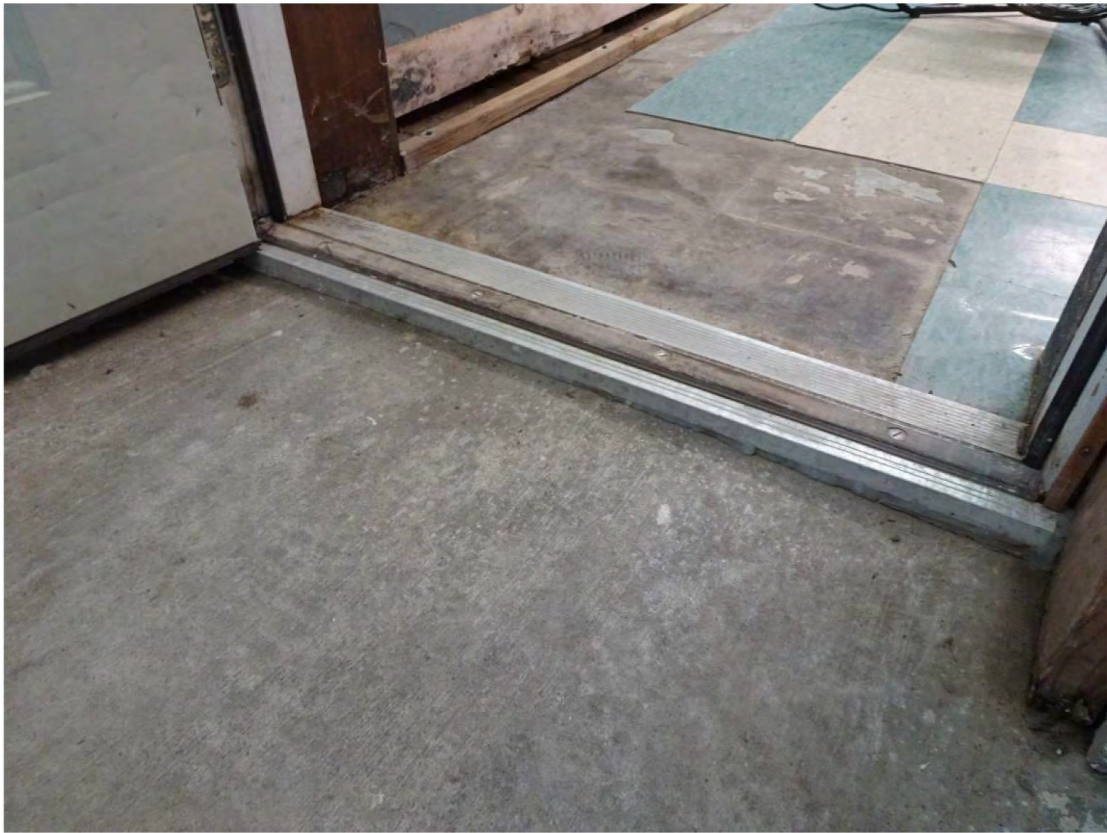
Non-Accessible Lower Level Ramp Threshold
